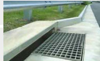
STORM WATER DRAINAGE & SEWERAGE LAID
