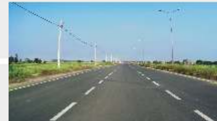
75M ROAD AND SECTOR ROADS READY
